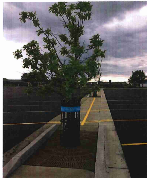
Tree trenches at Maplewood Mall
