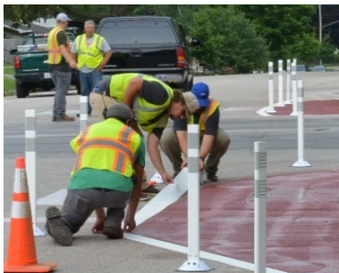
A temporary road project.
