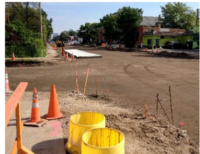
A road is reconstructed.
