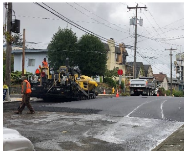
A road is resurfaced.
