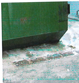
Dumpster Compactor Leaks
