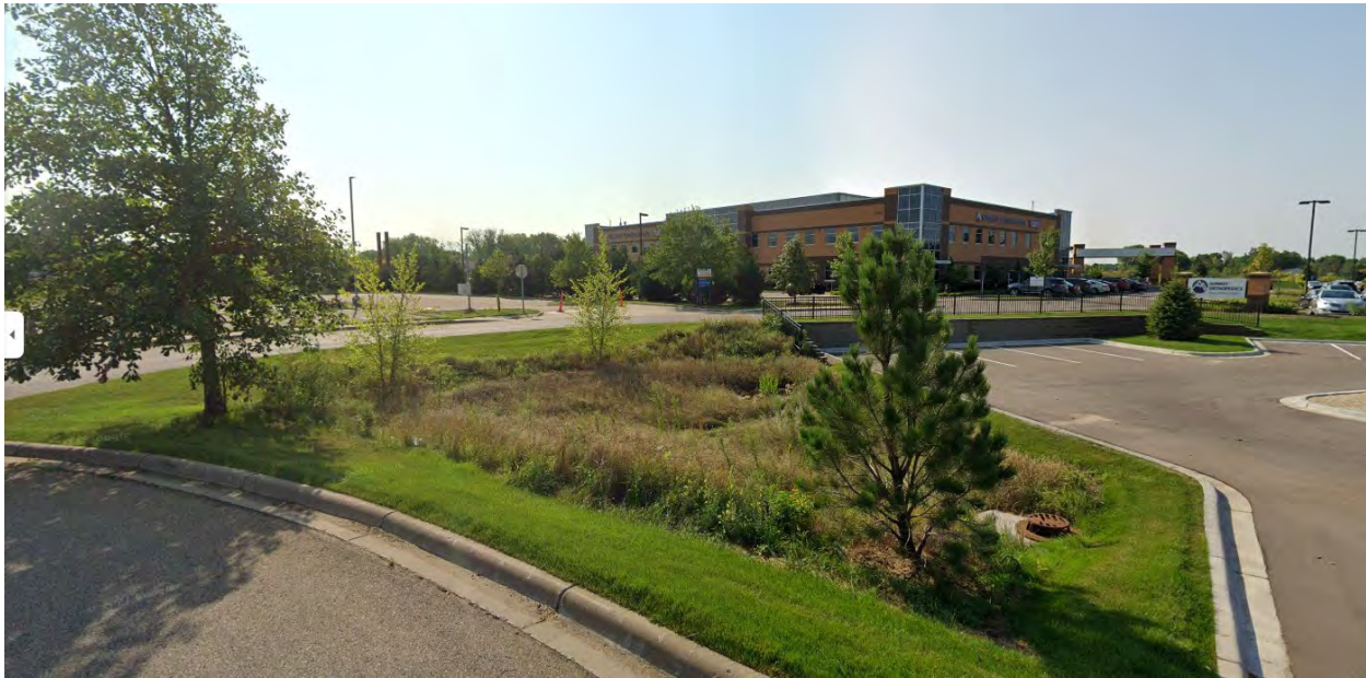
Figure 2- Biofiltration Basin with Trees
